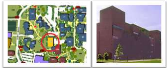
The newly-renovated Boggs Building now serves as the Nuclear and Radiological Engineering Department Headquarters
